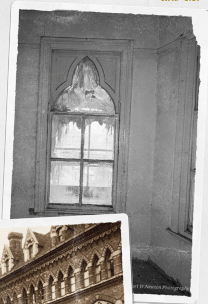
Interior Before Restoration (Below) Circa - 2020
